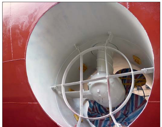
Thruster tunnel after application of first layer of Ecoshield.
