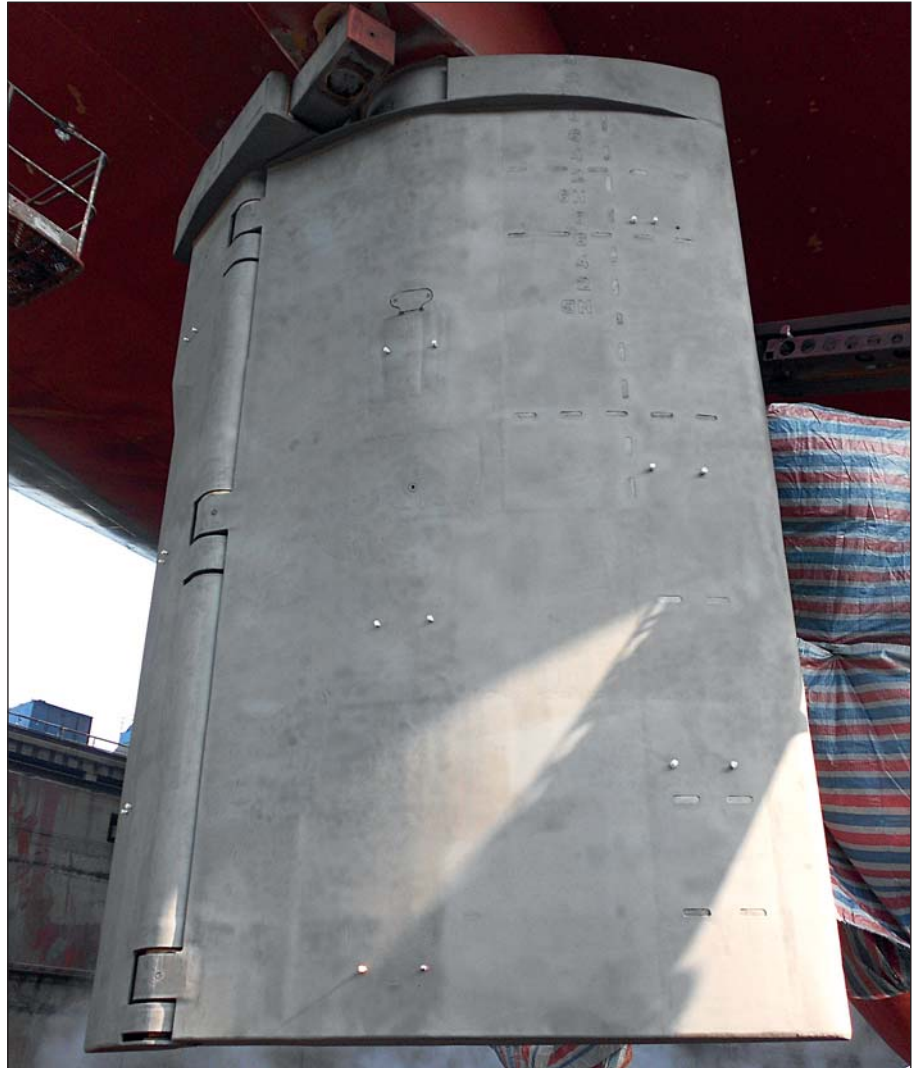
Rudder after surface preparation.
