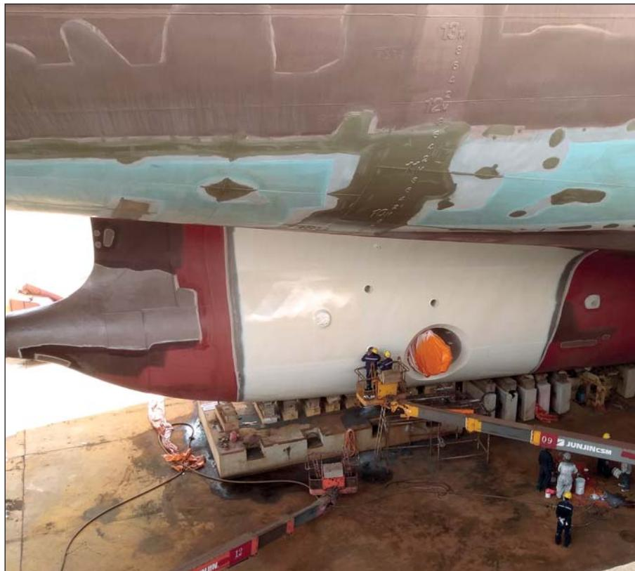
*Inspection of the scrubber outlet area after first layer.*
