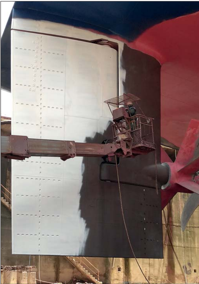
Ecoshield is applied in only two layers.
