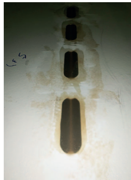
Slot welds filled with Ecofix.
