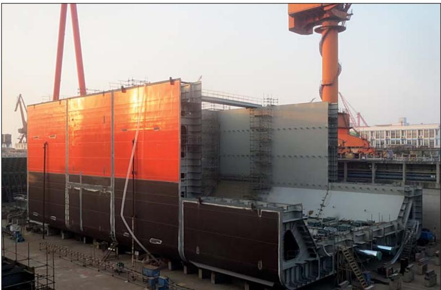
*Coating the weld seams after the blocks have been assembled is very easy and leaves a smooth finished surface.*
