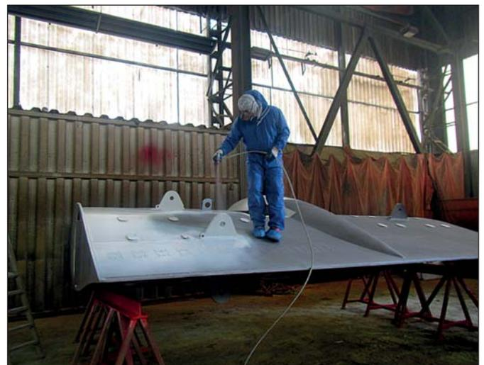
*Application of first of two identical Ecoshield layers.*
