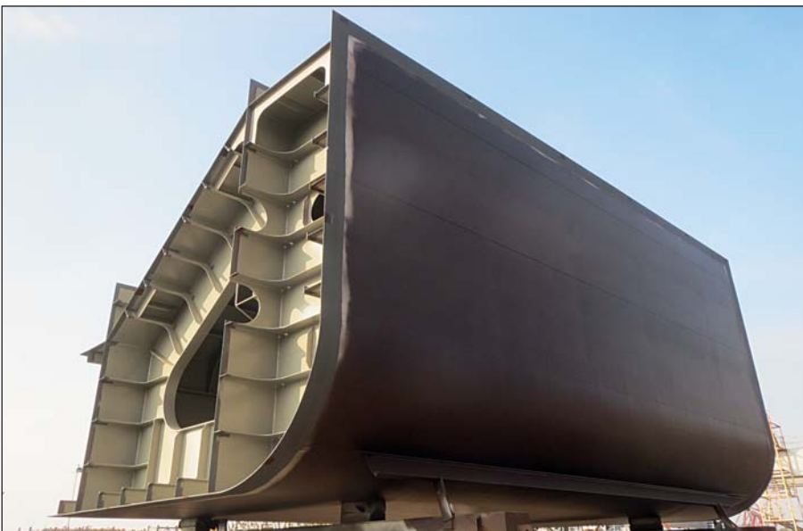
Finished application on one of the blocks of FSRU.
