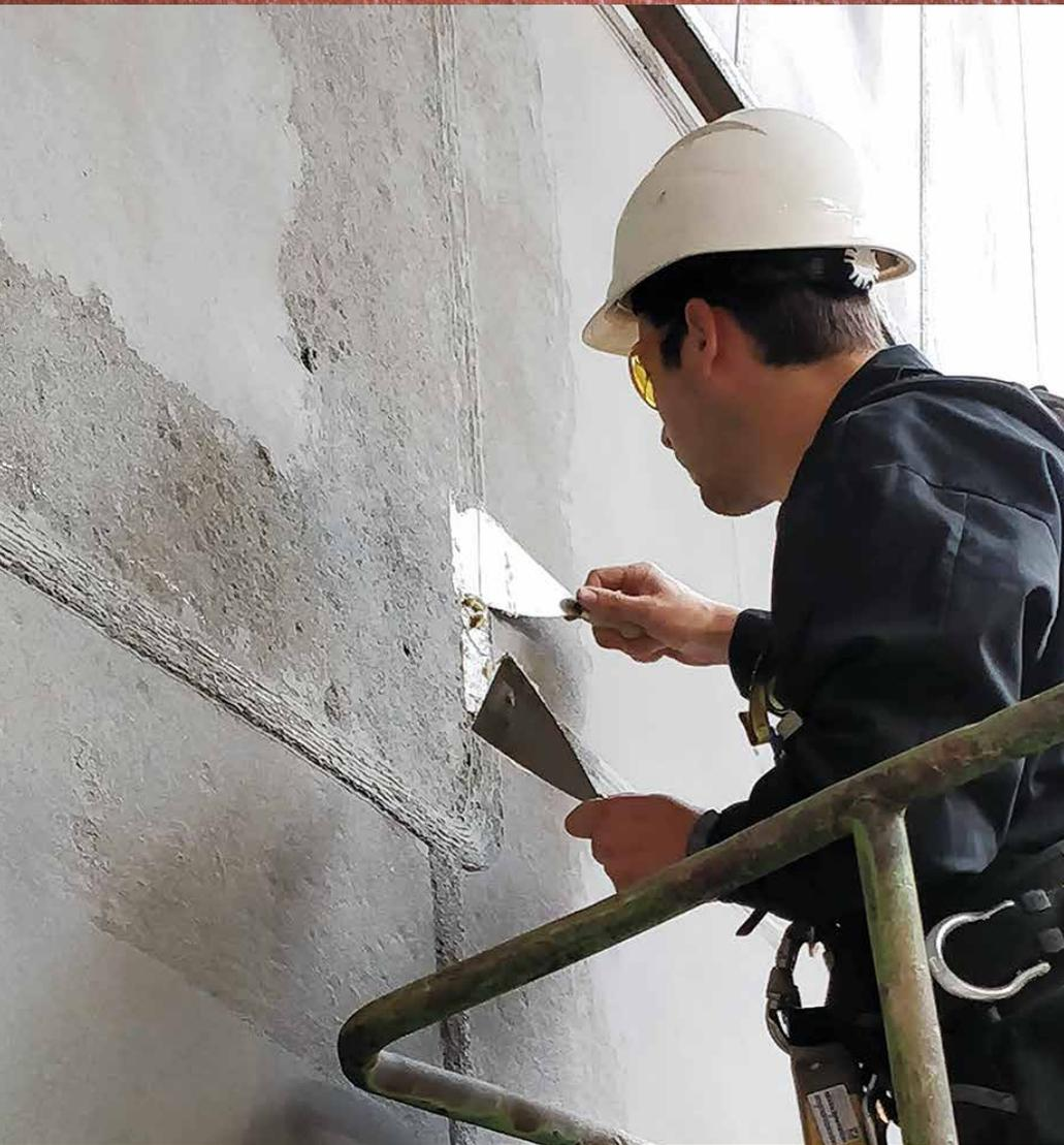
**E**cofix is a filler developed as a cost-effective solution for the repair of corroded or pitted steel surfaces prior to recoating with our coating systems.
