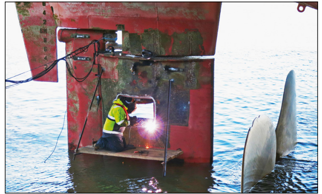
Rudder repairs in and out of drydock can be major expenses to a shipowner/operator.
