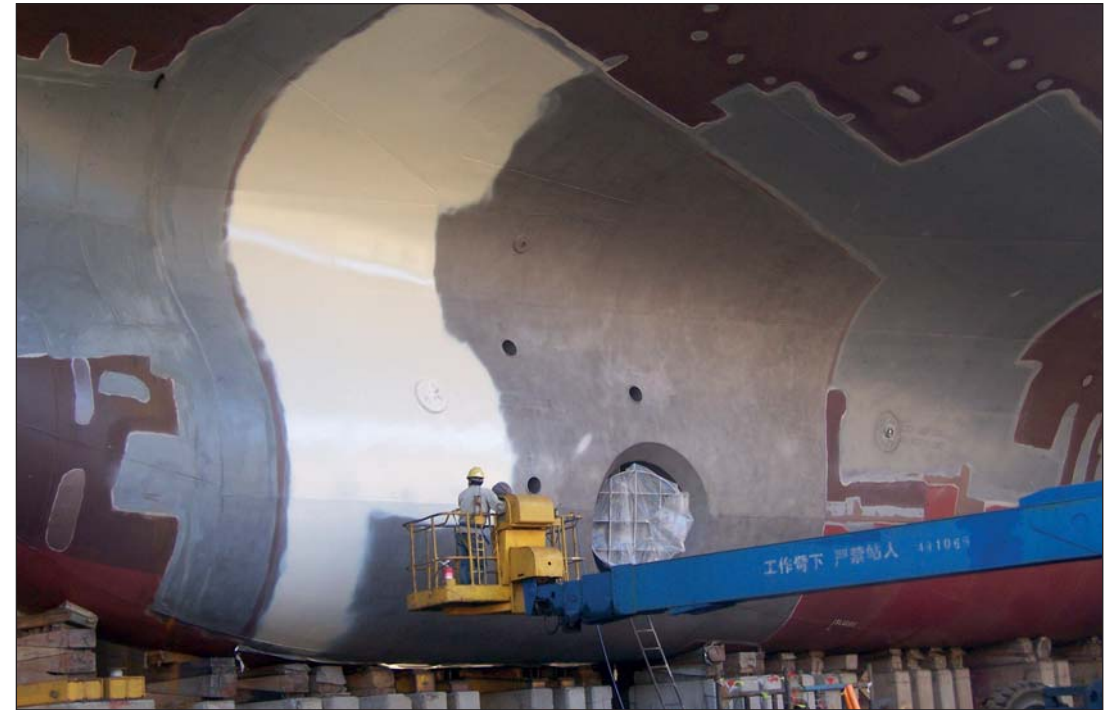
Application of first of only two layers of Ecospeed.
