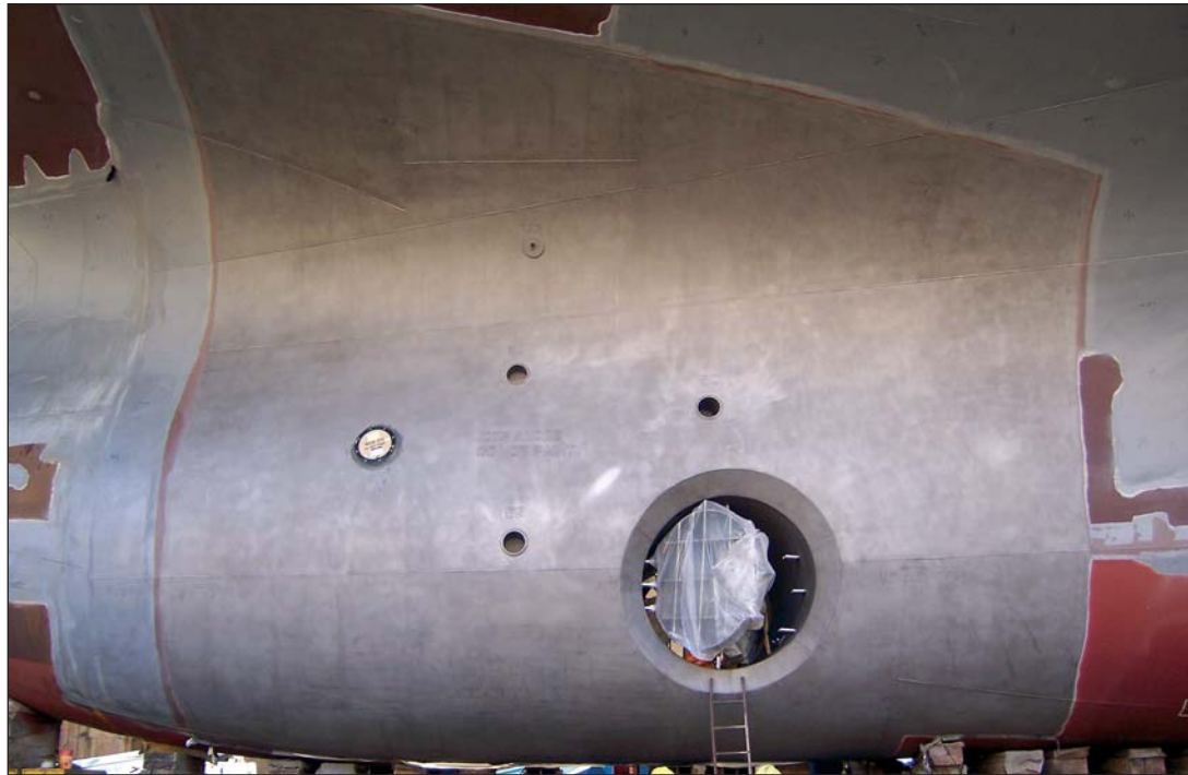
The area around the scrubber outlets after surface preparation.
