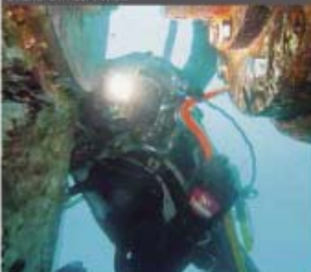
Underwater repairs by Hydrex on-board a tanker offshore West Africa
