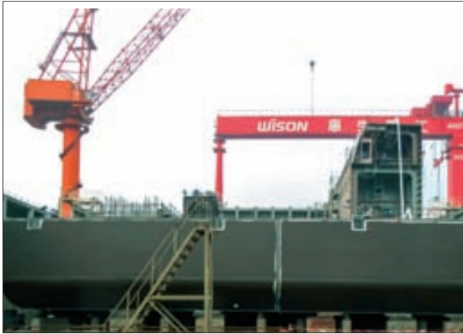
The Caribbean FLNG being assembled at the Wison shipyard
