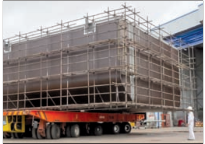
A fully coated block leaves the fabrication hall ready for assembly
