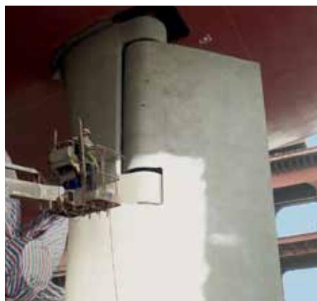
Good blasting preparation is vitally important before painting
