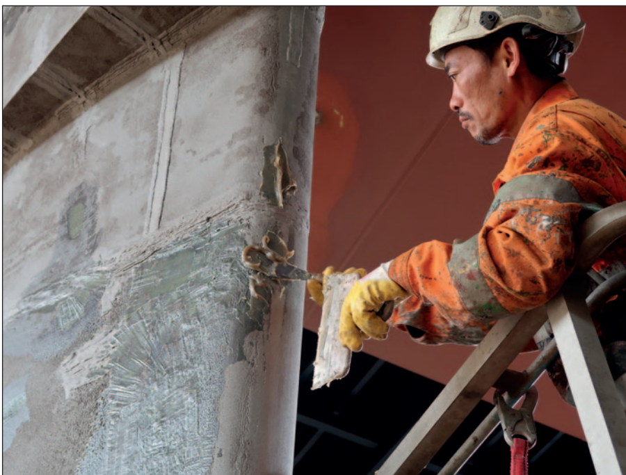
Application of Ecofix on corroded rudder.
