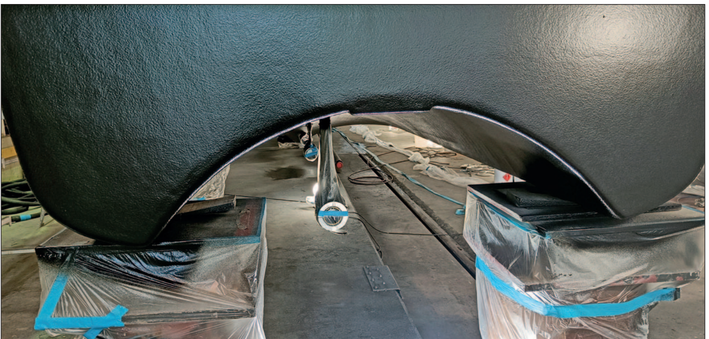
Hull of MS Brisen after application of both layers.
