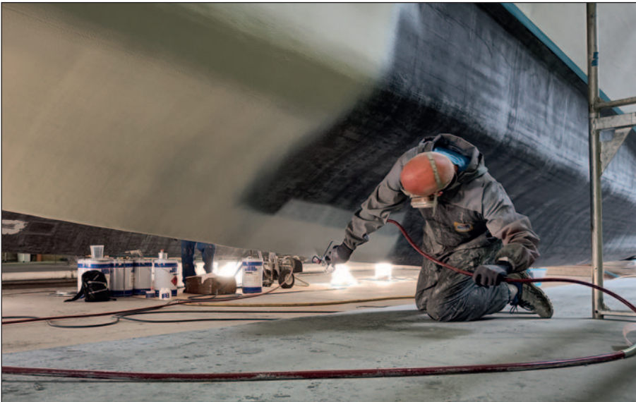
Application of first Ecospeed layer.
