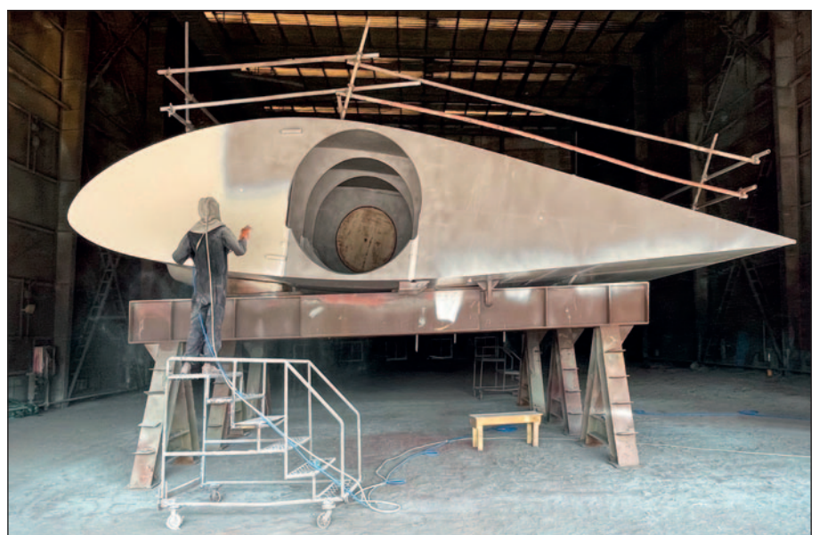
Application of first Ecoshield layer during the block phase.
