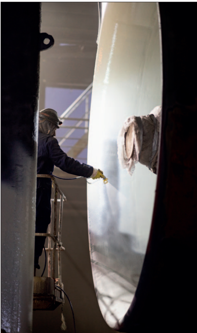
Application of first layer on propeller nozzle.
