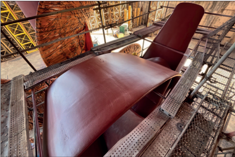
Stator fin after application.
