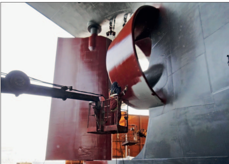
Second coat of Ecoshield being applied to a ship's rudder and Kort nozzle. This protection is expected to last the life of the vessel.
