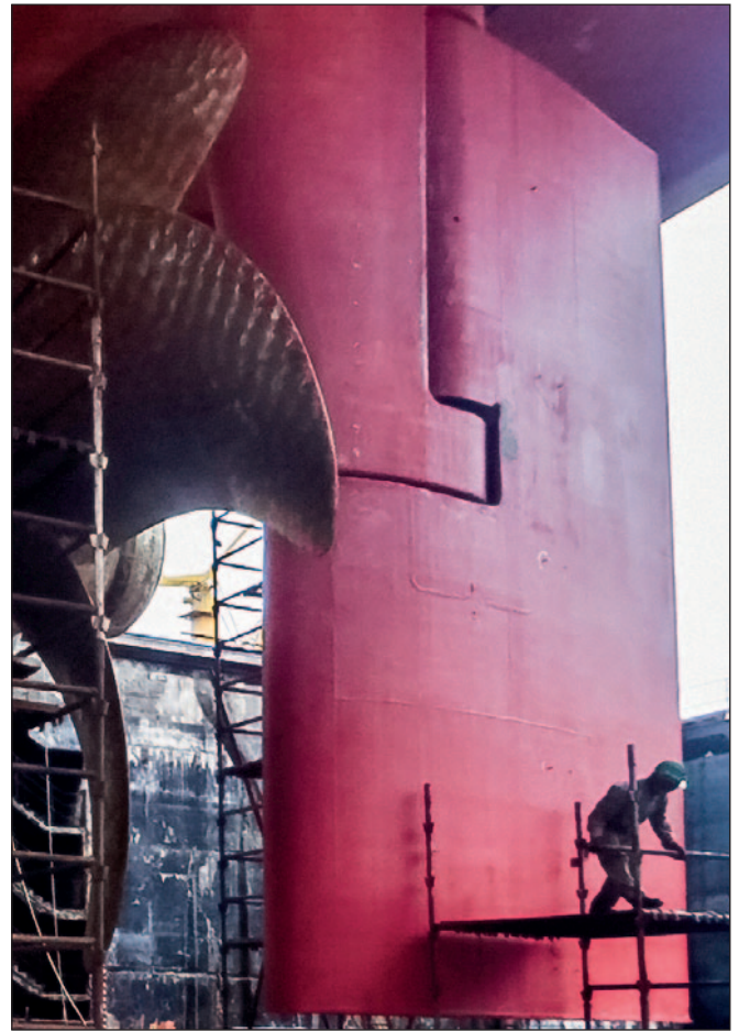
Danaos coated many of their rudders with Ecoshield. This is the Deva five years after the initial application, with no repainting.
