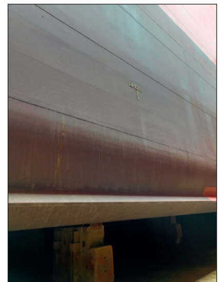
Ecolock coating in excellent condition 7 years after initial application, no repair or repainting, no cathodic protection.
