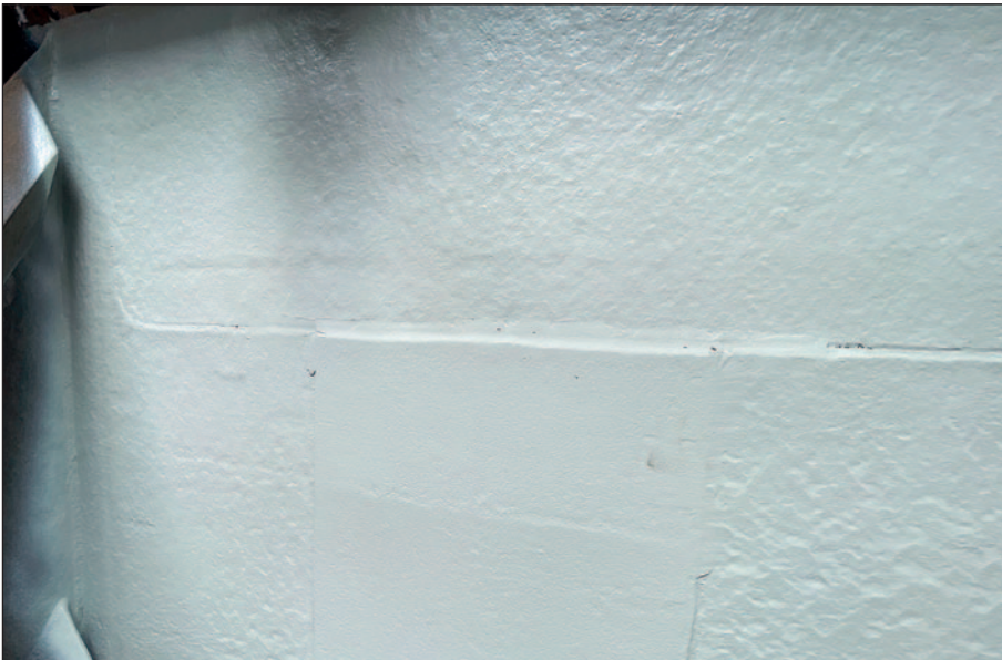
The first coat of Ecoshield applied.
