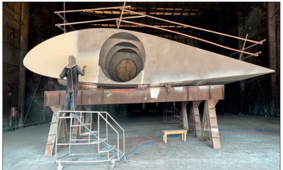
Application of first Ecoshield layer during the block phase.
