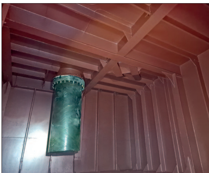
Recycle tank protected with Ecospeed.
