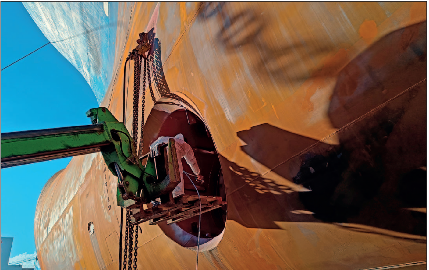
Ecoshield application on thruster tunnel.
