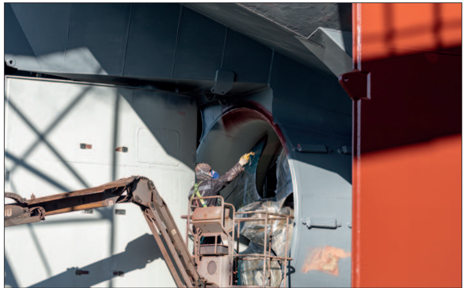
Application of second Ecoshield layer on propeller nozzle.
