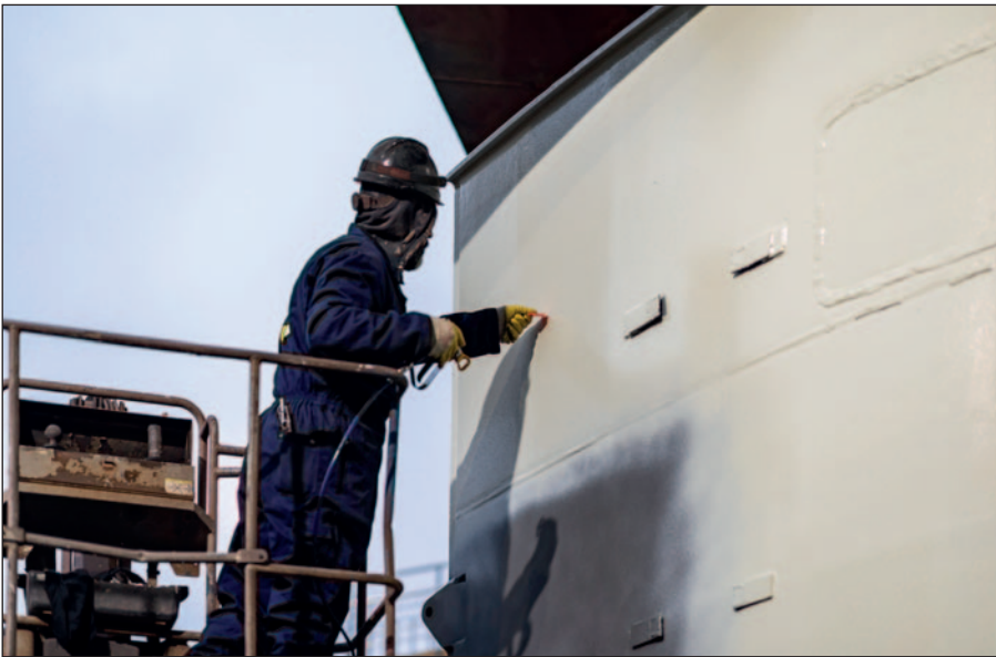
Paint applicator measuring the wet film thickness during application.
