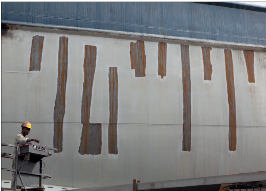
Ecospeed coated hull where hot work inside the ship has damaged the coating.
