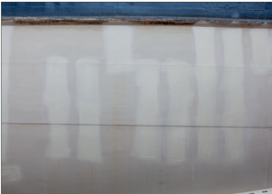
The damaged Ecospeed coated hull repaired, leaving the hull as smooth as when first painted.
