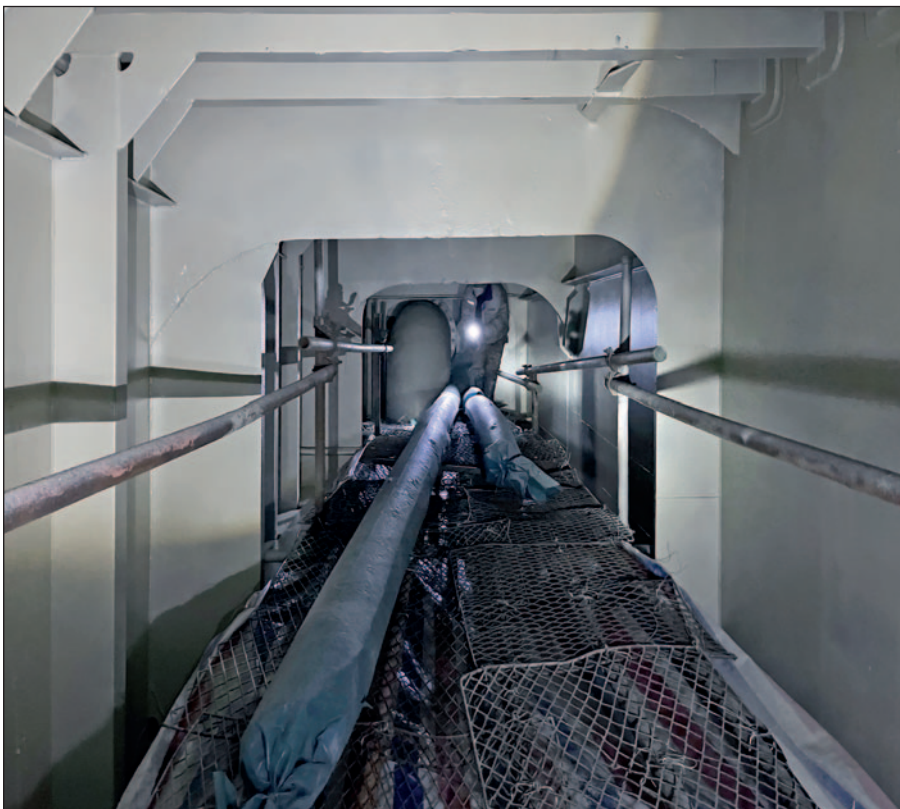
Recycle tank after application of first Ecospeed layer.
