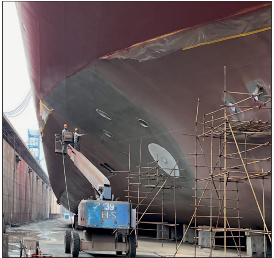
Ecospeed application on scrubber outlet.
