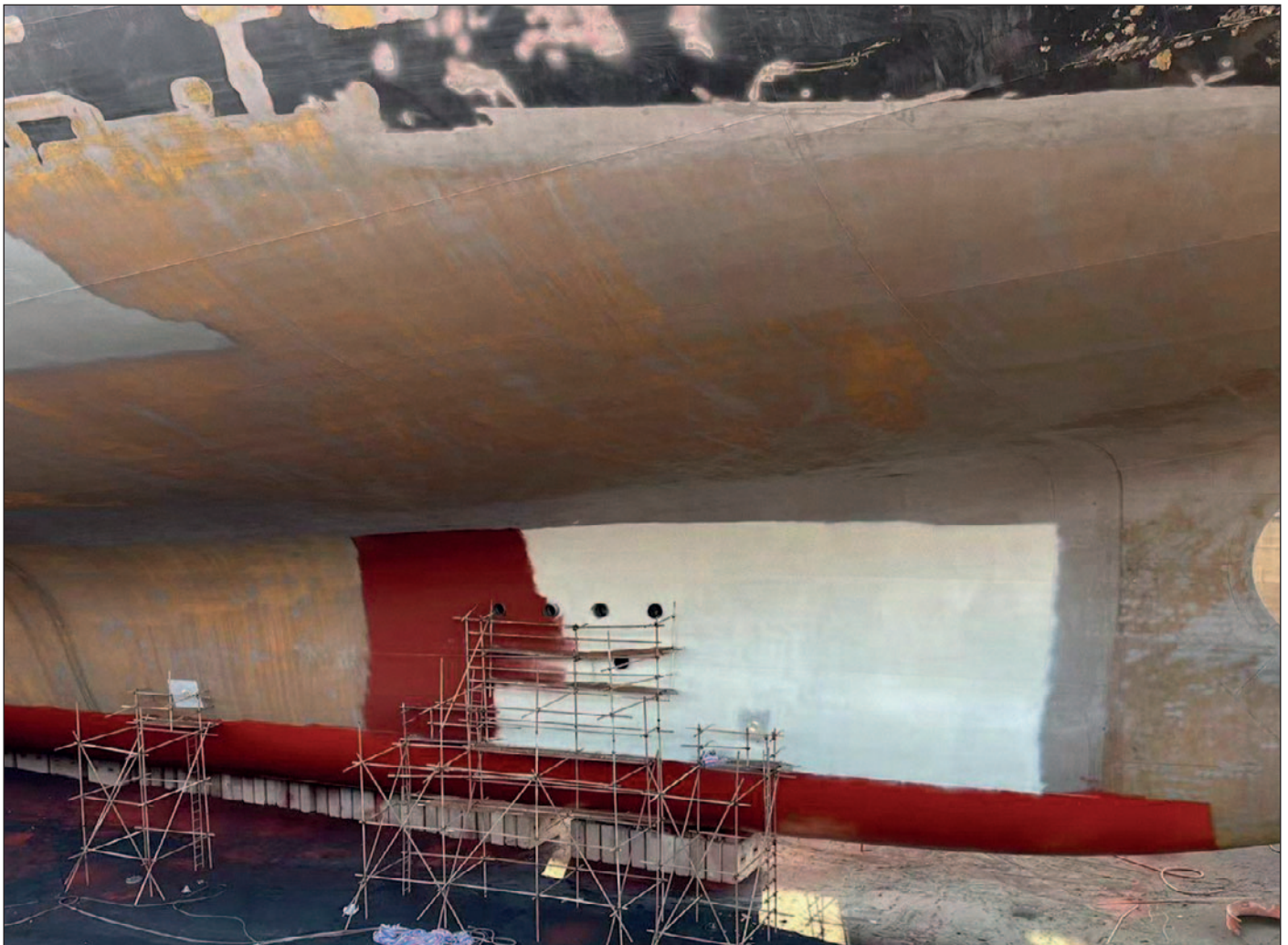
Ecospeed is applied in two identical layers.
