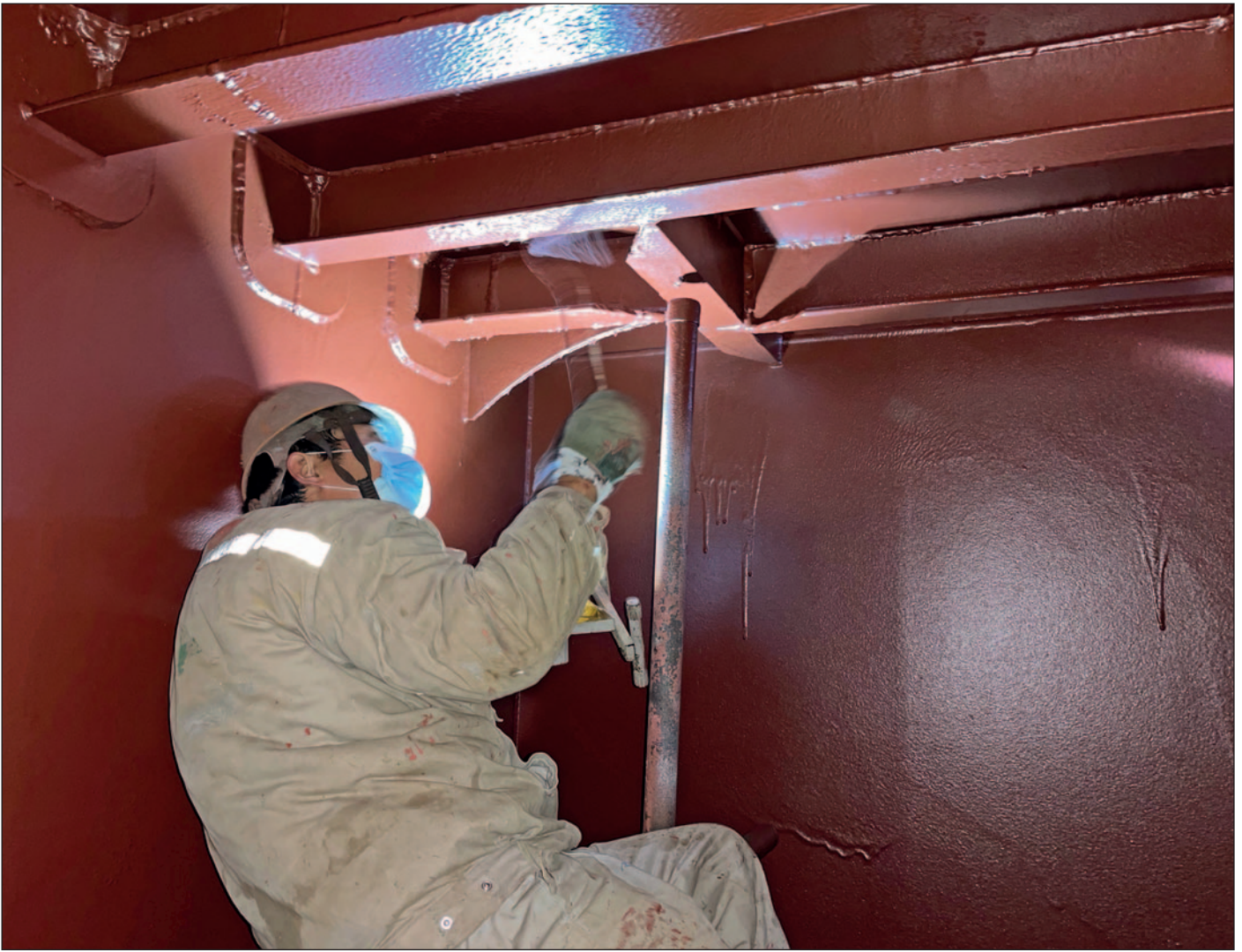
Application of second Ecospeed layer in scrubber tank.
