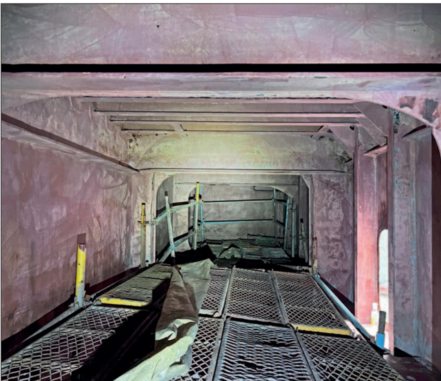
After two years of chemical residue passing through, the Ecospeed coating is still in excellent condition and has protected the steel from corroding.
