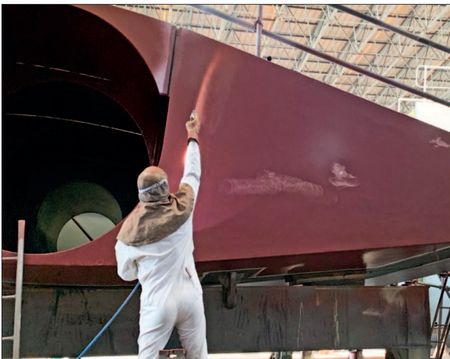
Ecoshield being used at the newbuild stage to provide lifelong protection to a rudder.
