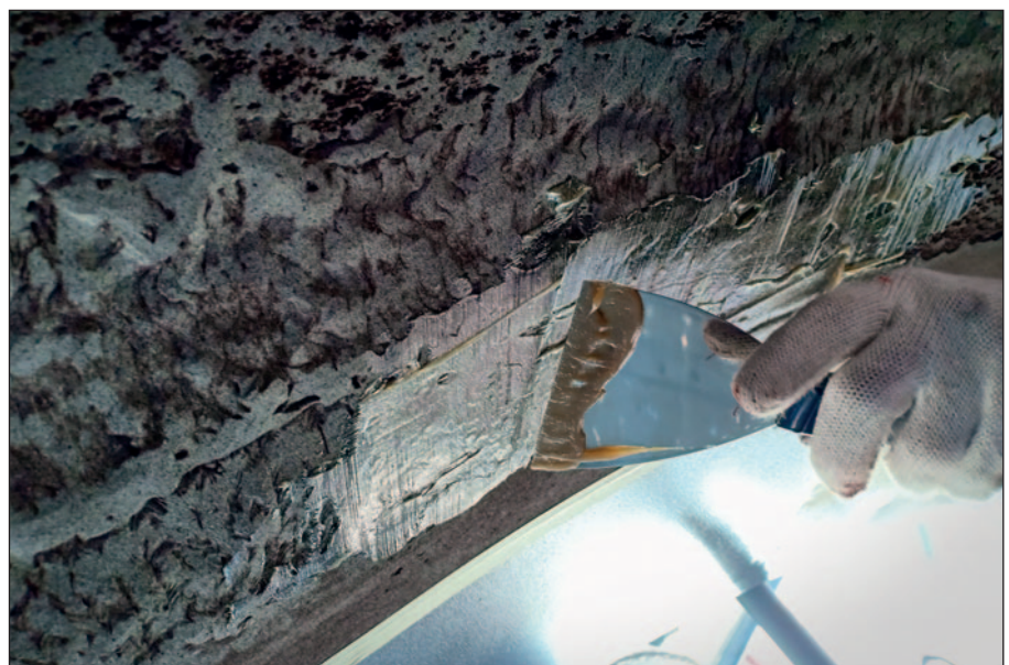
Ecofix is a filler which is compatible with Ecoshield and used to repair pitted surfaces prior to Ecoshield application. Overcoat time is 1 hour.
