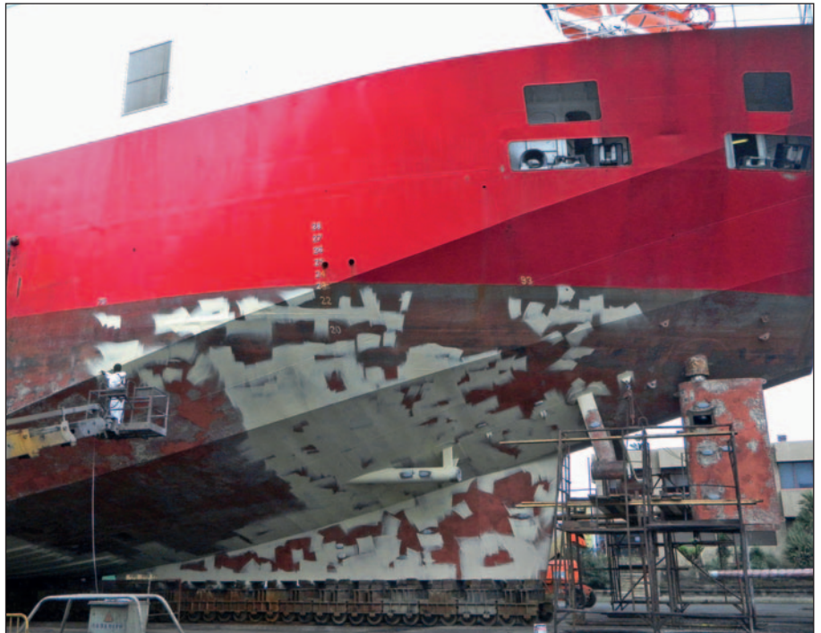
Typical repair in drydock of an antifouling coating which is patched and then a new topcoat applied.
