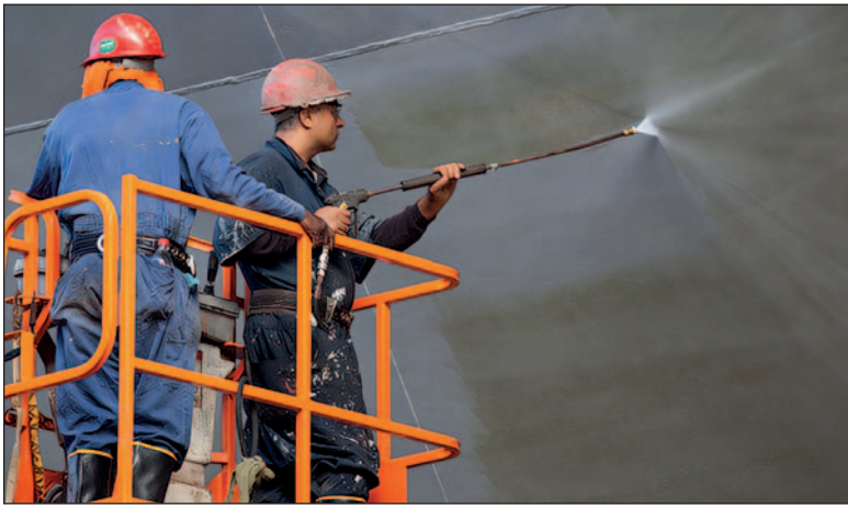
High pressure washing in drydock is very effective in cleaning Ecospeed.
