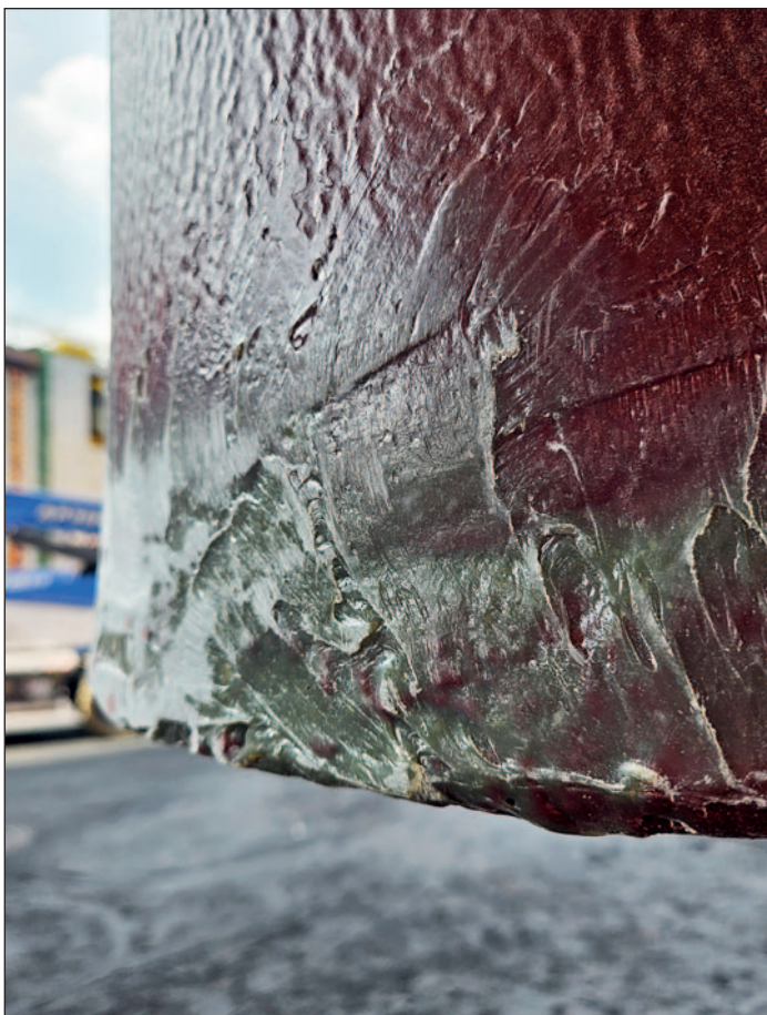
Ecofix is a filler which is compatible with Ecoshield and used to repair pitted surfaces prior to Ecoshield application. Simple, fast, and low cost.
