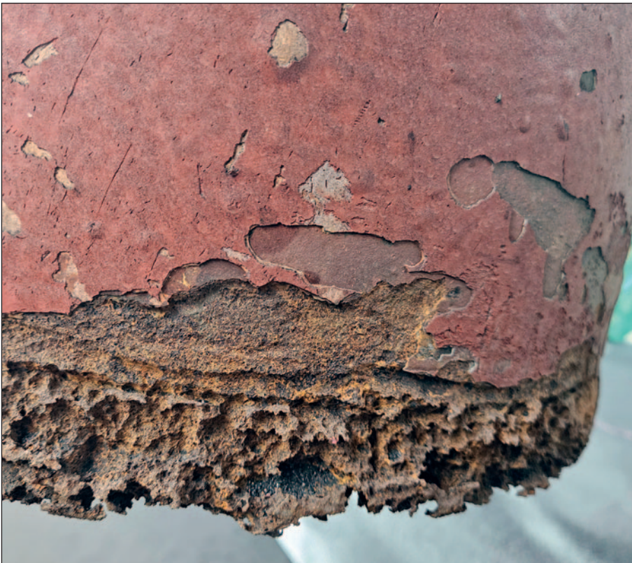
Severe pitting on rudder as a result of cavitation. Ecoshield can prevent this from happening again.
