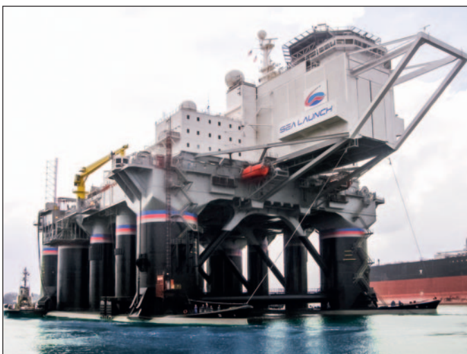
The Odyssey's hull after grit blasting and recoating.
