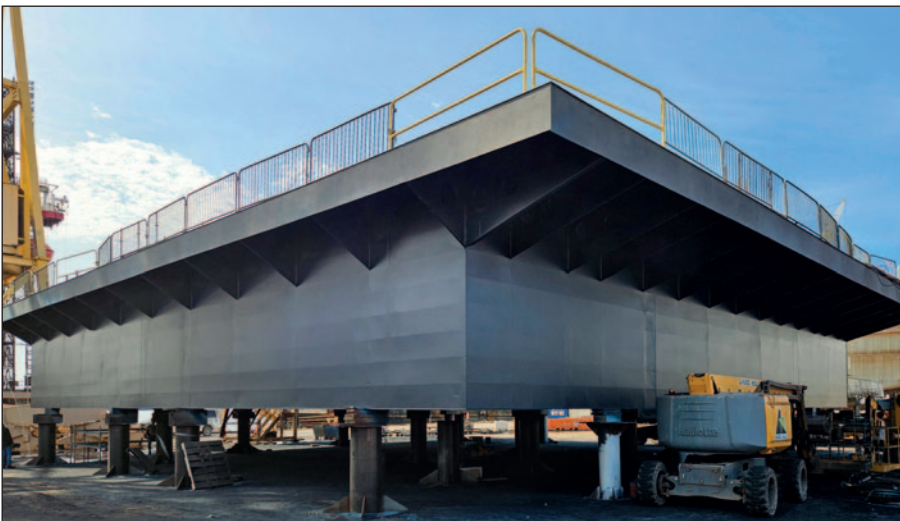
Our coatings are a perfect fit for a wide range of projects, like the underwater structure of a floating pool in New York.
