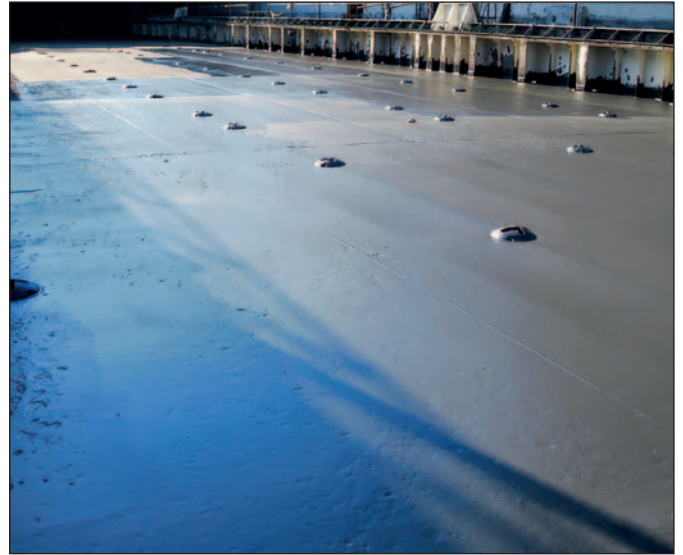
The deck after Ecospeed application.
