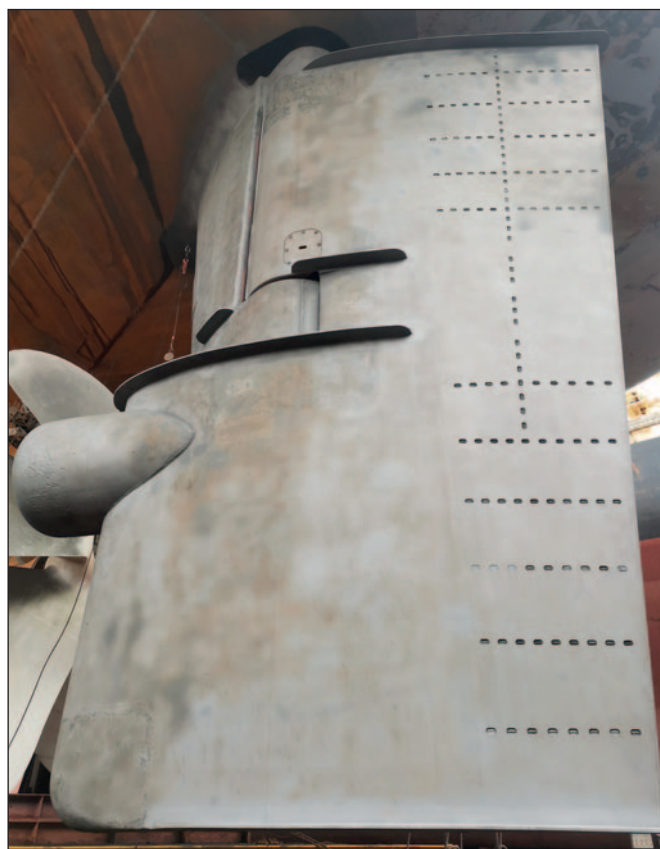
Rudder after surface preparation, ready for Ecoshield application.
