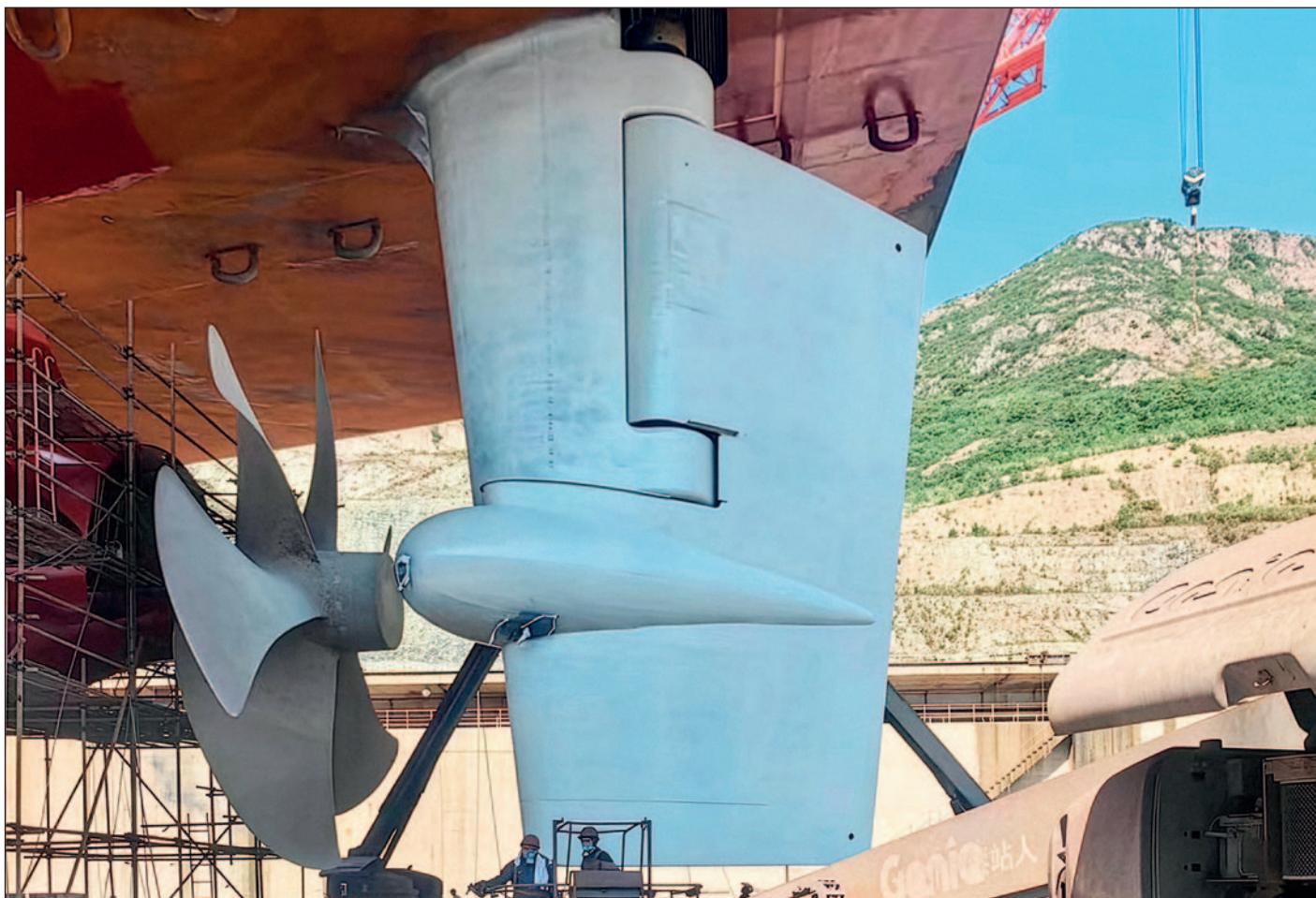
Rudder after application of first Ecoshield layer.
