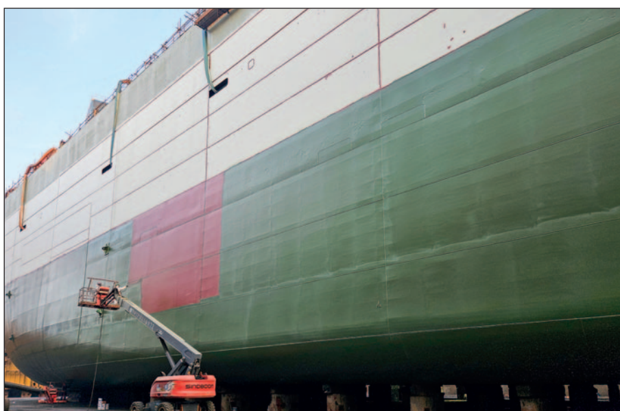
One of two LNG carriers converted to FSUs to be stationed offshore in British Columbia, receiving the third coat of Ecolock (green) on the underwater hull.
