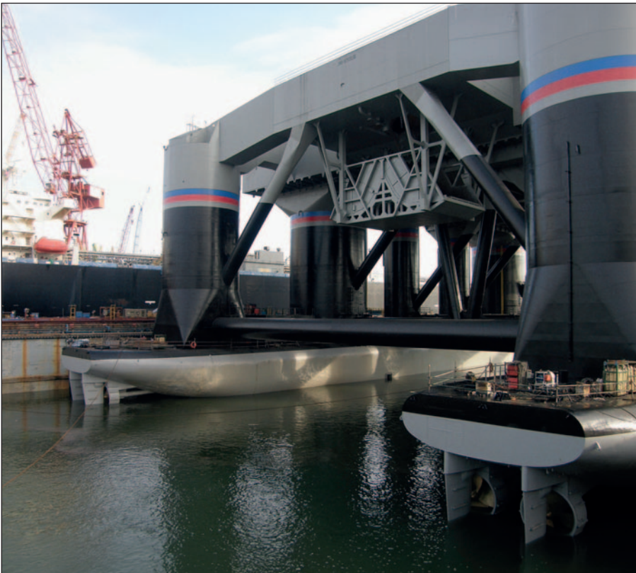
The Sea Launch Odyssey semisubmersible rocket launch platform at its home port of Long Beach, California. The hull is protected with Ecolog.
